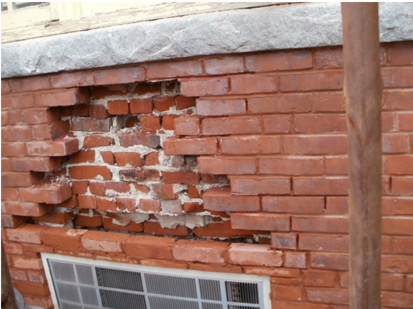
Entire Sections of Brick Collapsed During Masonry Repointing During Phase I (Building Exterior Adjacent to Bill's Pizza)
