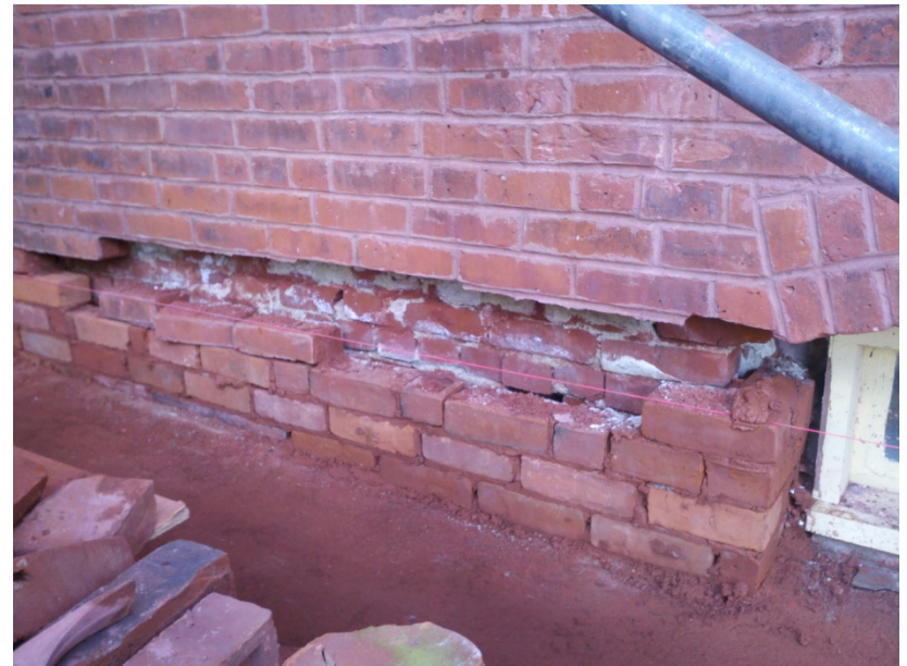
Entire Sections of Brick Collapsed During Masonry Repointing During Phase I (Building Exterior Adjacent to Bill's Pizza)
