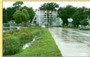
Bioswales are rain gardens that run parallel to streets and infiltrate stormwater. Photo courtesy of Natural Resources Conservation Service.
