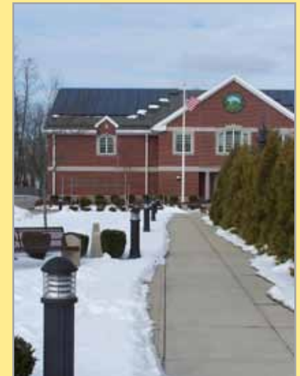
Hopkinton's police building recently installed solar panels and reduced their dependence on traditional energy.
