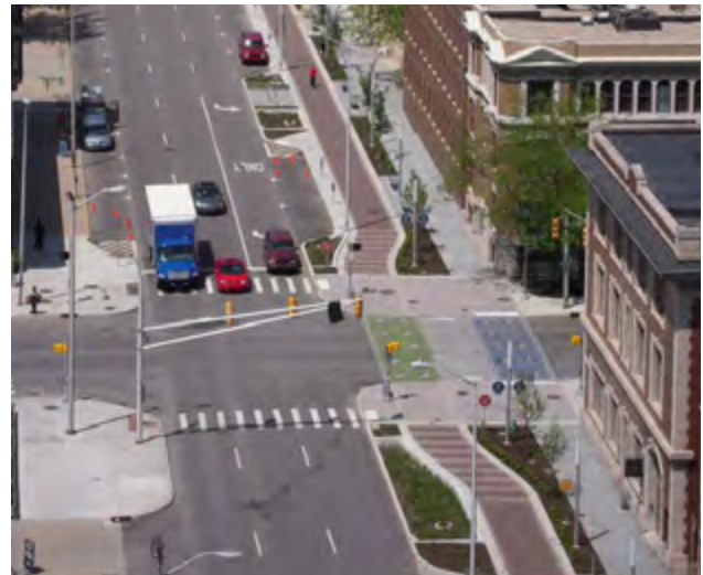
The Cultural Trail in Indianapolis uses rain gardens to collect and filter stormwater runoff, incorporates tree plantings, allows on-street parking to buffer trail users from the street, and clearly marks intersections for pedestrian and bike crossings. (photo: Rundell Ernstberger Associates)
