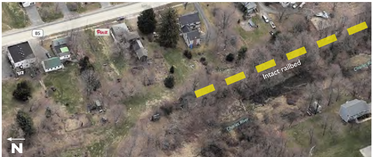
Portions of the railbed between Granite Street and Chamberlain Street have been demolished or built over in places, as is the case here. Houses sit especially close to the railbed in this segment; its ownership is divided between fifteen separate property owners (photo: Bing BirdsEye).
