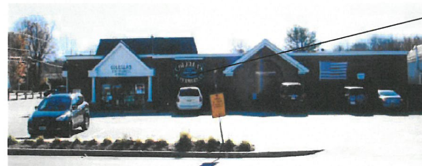
C Photo Comp - Existing North Elevation Not to Scale
