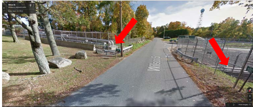
Figure 1. Image of the pipeline road crossing under Wilson St. at the NSTAR facility. Note that any LNG spill from the pipeline will collect in the depression on the right side (west) of the road. Arrows indicate the pipeline impact point identified by Smith & Burgess and the depression.
