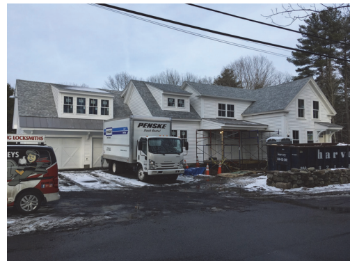
Work in progress at 26 Fruit Street
