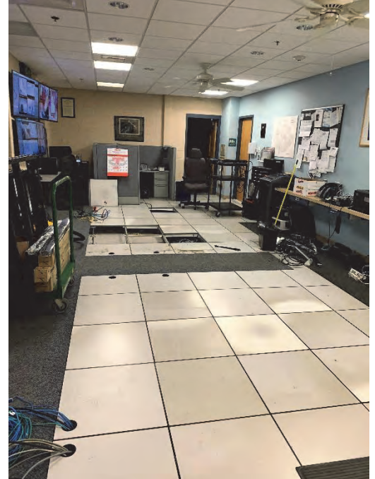
Right: Old workstations have been removed. Underfloor wiring was reorganized to prepare for the new consoles. Broken floor tiles were removed and replaced. All floor tiles were reassembled and prepped for the new workstations.
