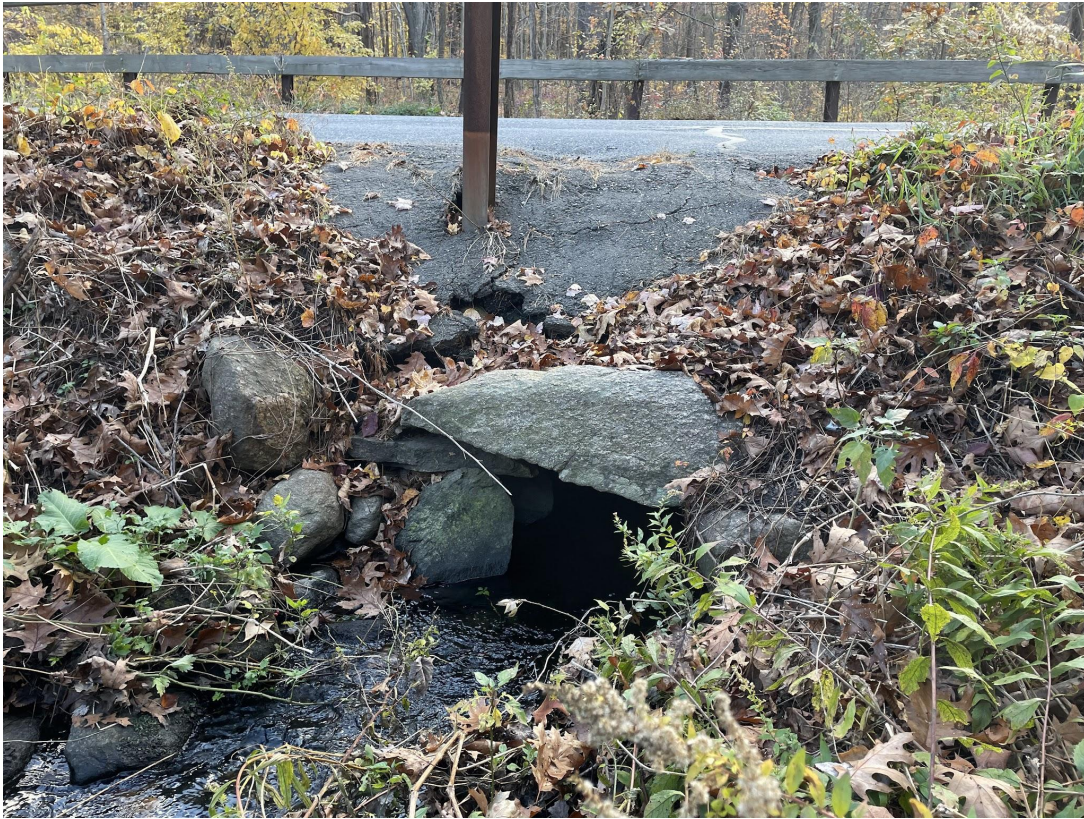
Photo 1: Granite Street culvert, on south side of Granite Street looking north
