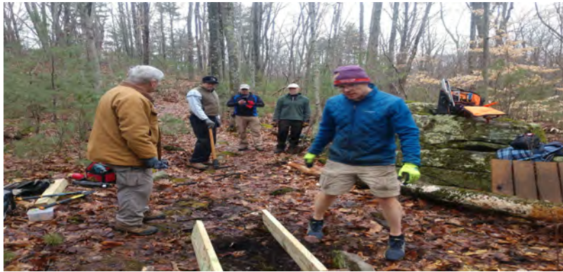
(Bridge construction at Cameron Woods)
