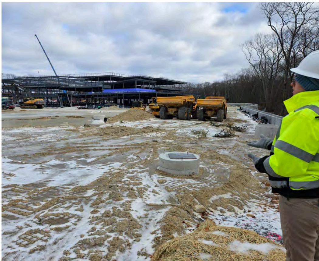
(Above) Staff inspect the Charleswood School construction site
